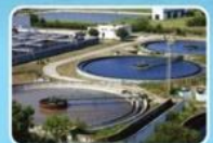
Sewage treatment plant rehabilitation & development
