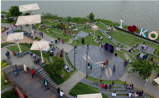
Public space (above) around the lake developed using a combination of natural grass and semi-pervious paverblocks
