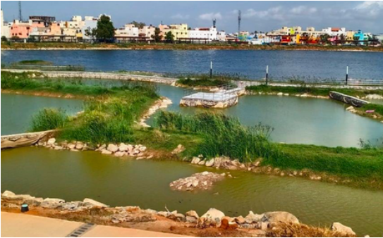
Selvachintamani Wetland (above) developed to treat primary and secondary treated used water from drains and the treatment plant naturally before the water flows into the lakes. Seasonal flooding fertilises soil, and terraced landforms serve as a natural stormwater management infrastructure
