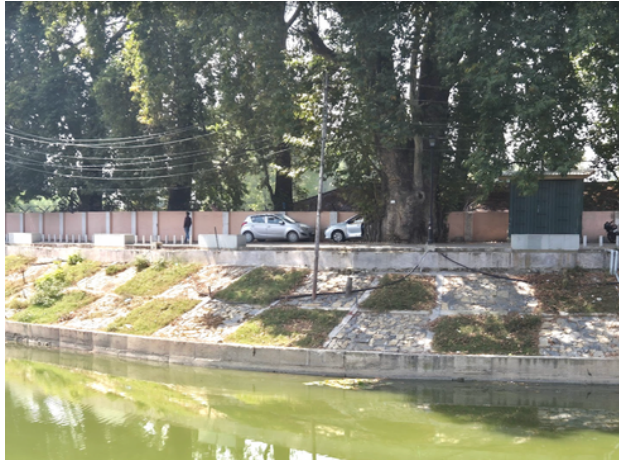
Vegetated rip-rap bank treatment on the interconnected water channel of Jhelum to maintain the natural interlinkages within the ecosystem
