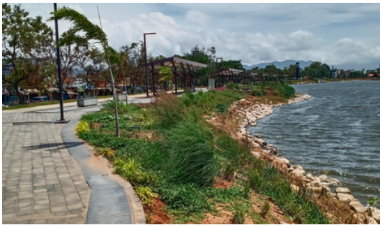
Sloped water-edge planting using native species to improve biodiversity and absorb sudden shocks
