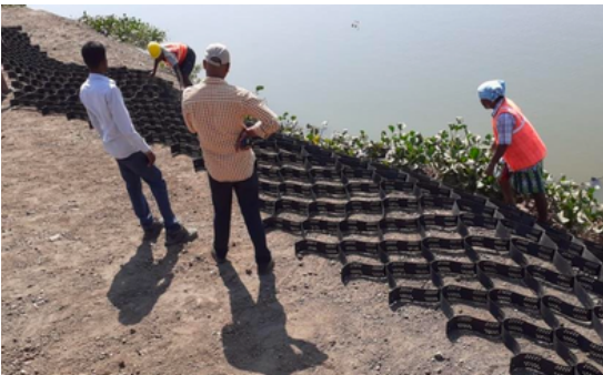
Bund strengthening (above) using ring bunds and native plantation for improved resilience at lake edges
