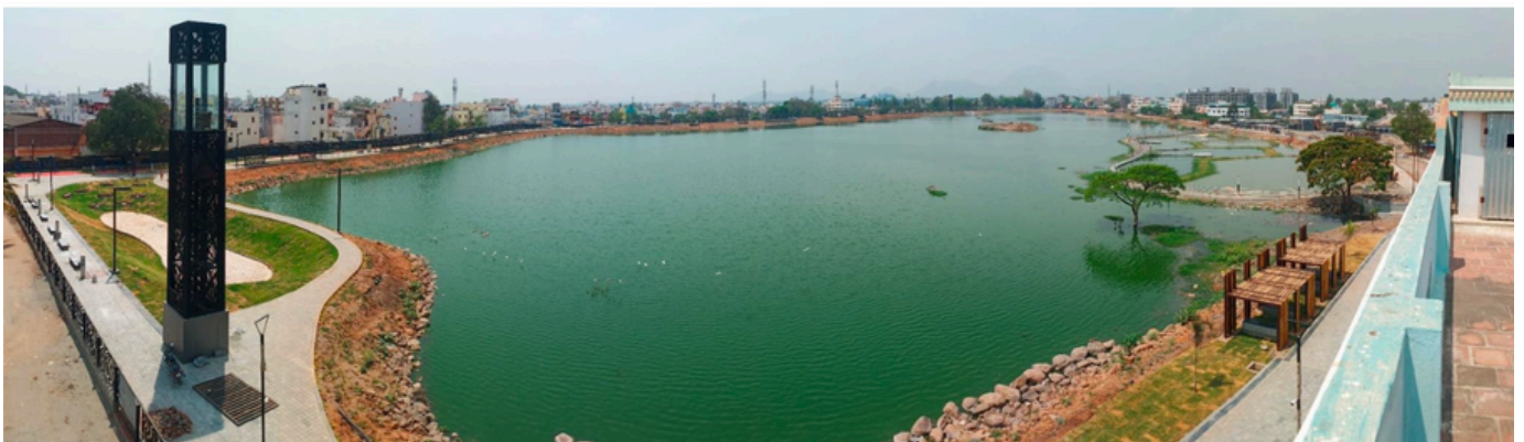
Restoration of lake and its edge (above) integrating native plantation and rocks on sloped edge, with cycle lanes as public promenades
