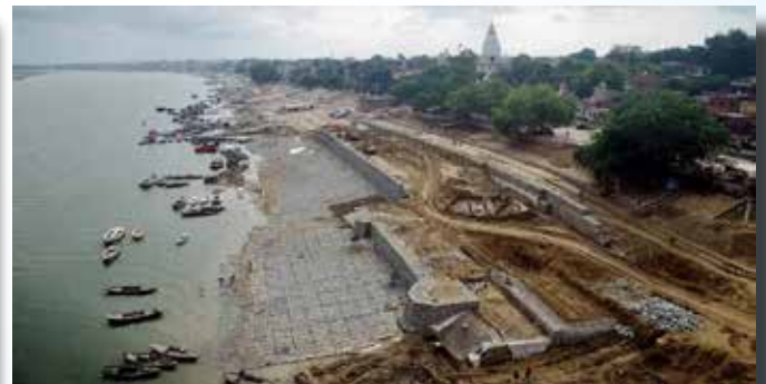
Figure 4: Kashi Vishwanath Corridor Under Construction
