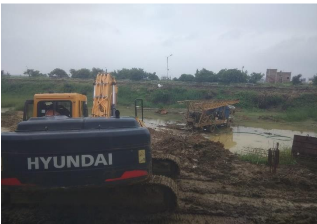
Construction work – Pahari STP
