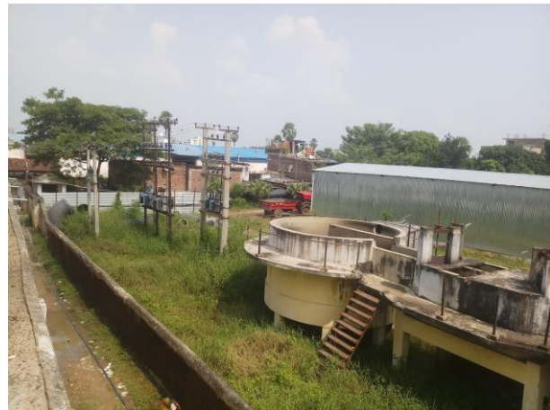
Existing STP at Pahari
